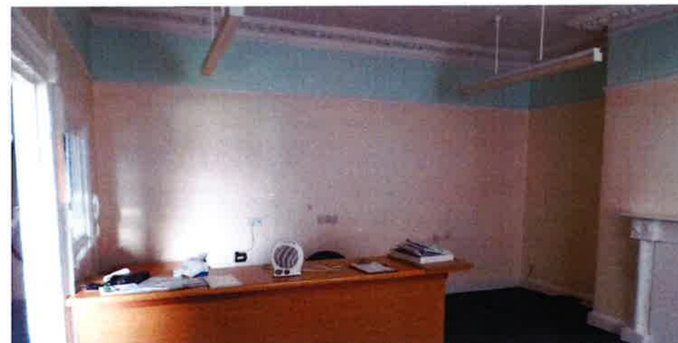
1 Beach Road: Retained feature windows, stair ceiling cornices and door architraves
