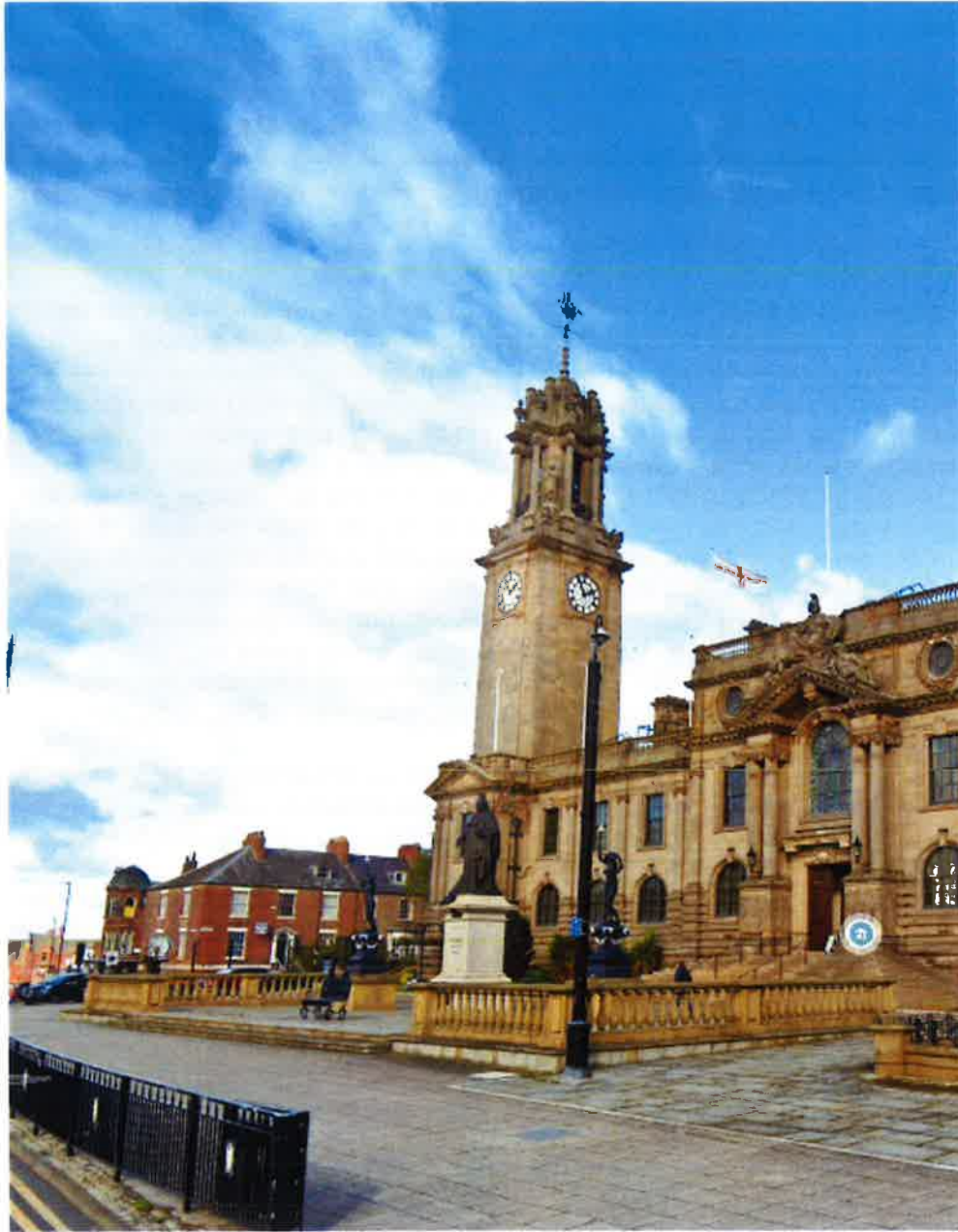
Beach Road setting backdrop to Town Hall
